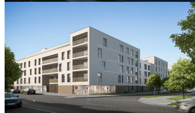
Pierreries 82 logements + rez commercial Rue Emile Delva, 1020 Laeken Antonissen Development Group Compromis : 2020
